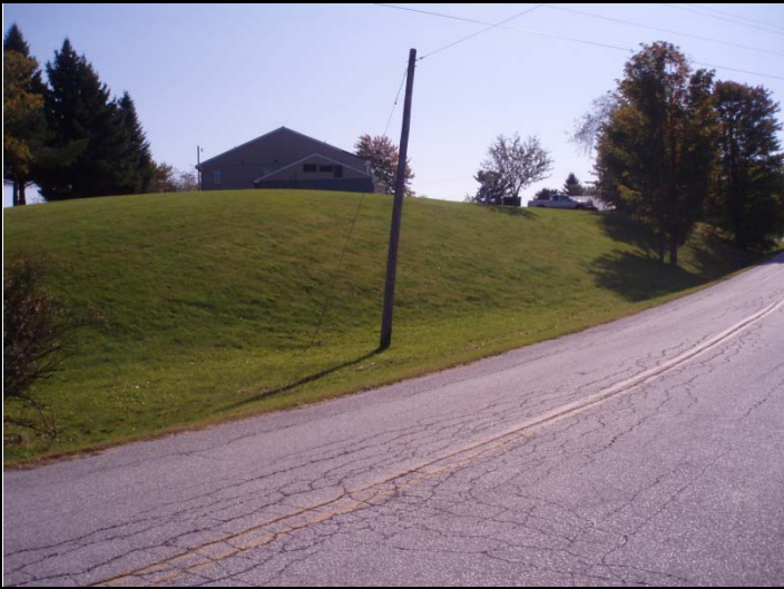
Photo 1. Overview of potential area, existing drainage
