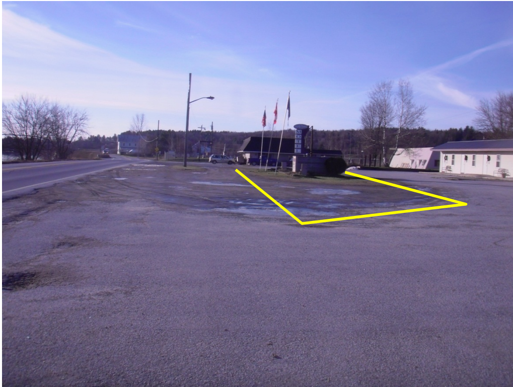
Figure 5. A stormwater treatment practice in the parking median at the Dairy Center could be an effective option with minimal impact on the parking lot traffic patterns.
