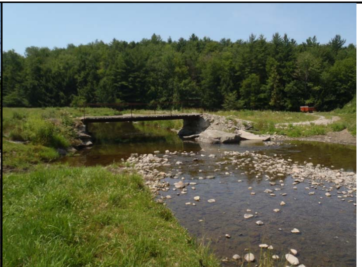
Photo 2. Farm crossing in reach
