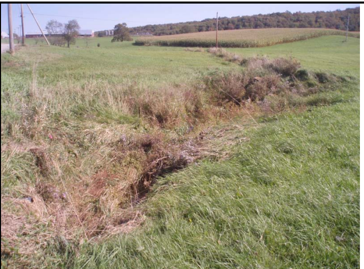
Photo 2. Ditch near the Miss VT Dr, on Howrigan Rd
