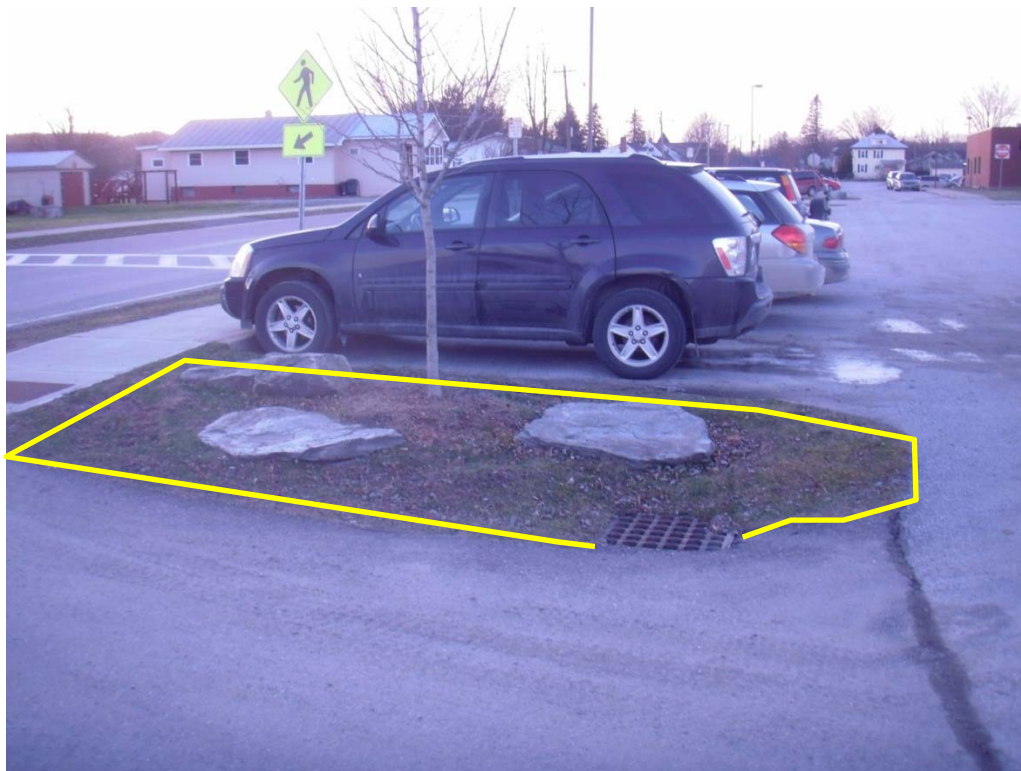
Figure 14. This parking island could be utilized to treat stormwater with a simple retrofit design creating a small bioretention basin.
