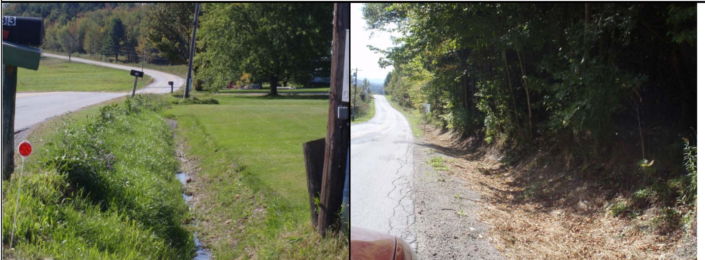
Photo 1. Ditch along Water Tower Rd
