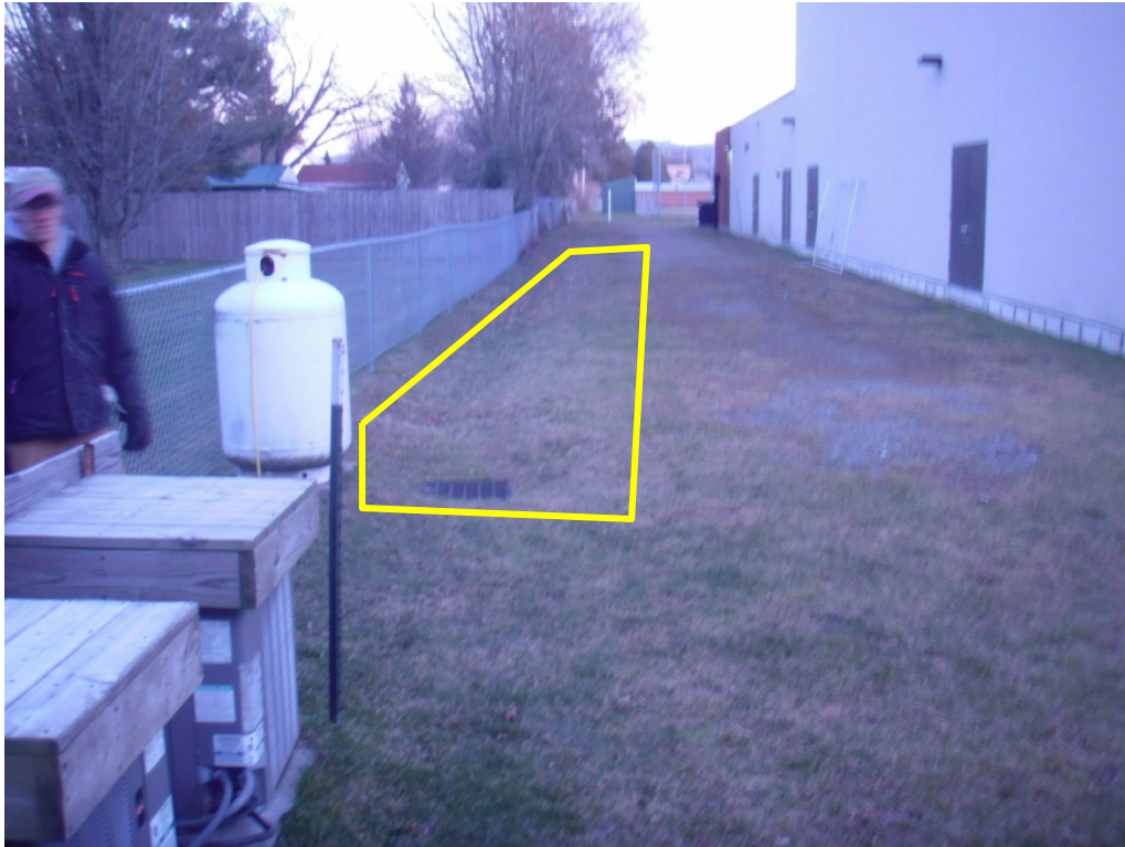
Figure 12. A catch basin to the rear of the high school could easily be retrofitted with a stormwater STP such as a bioretention swale to capture and detain roof runoff.
