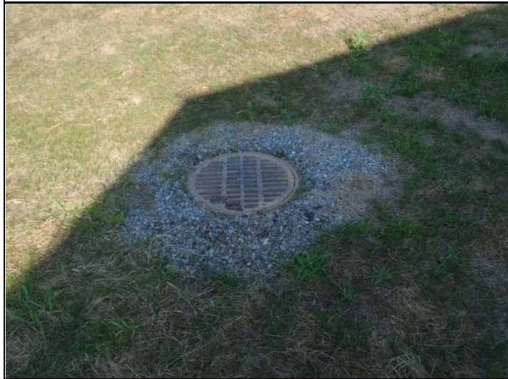
Photo 1. Catch basin outside of WW plant
