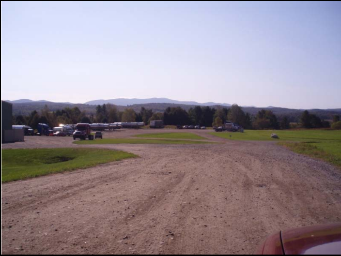
Photo 1. Overview of Industrial Park development
