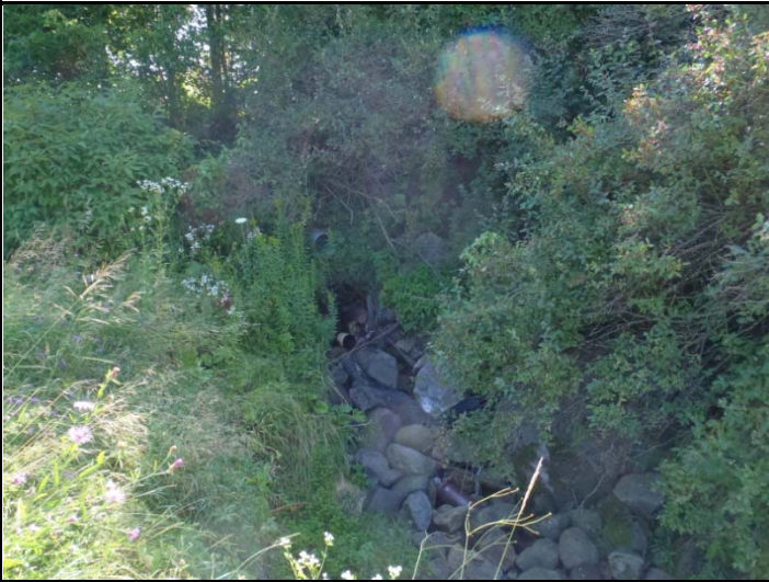
Photo 1. Outfalls and rip rap
